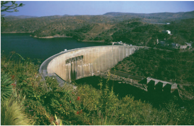
Figure 5.2 The Kariba Dam on the Zambezi River between Zambia and Zimbabwe. Such large dams can provide protection against floods and water shortages, and generate a great deal of electricity. However, they can have a whole suite of environmental consequences. (See Plate 33)
