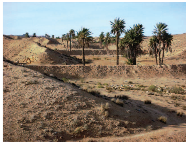
Figure 4.16 Soil conservation banks across a small ephemeral channel (wadi) in the Matmata area of Tunisia. (See Plate 31)
