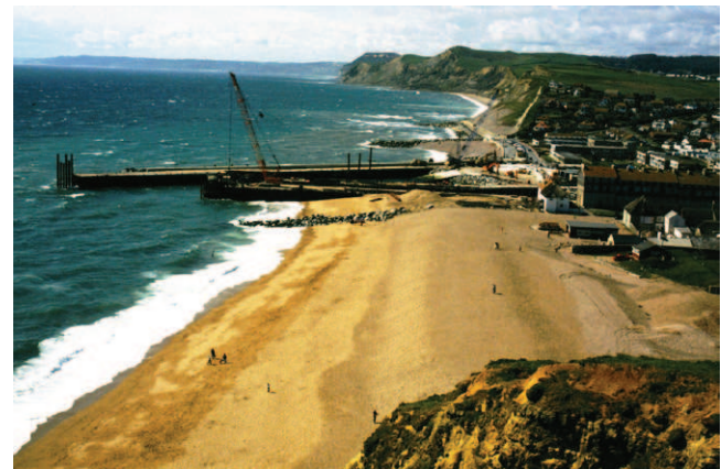
Figure 6.27 In the nineteenth century a jetty was built at West Bay, Dorset, southern England to facilitate entry to the harbour. By the twenty-first century accretion has taken place in the foreground and erosion in the background. (See Plate 44)
